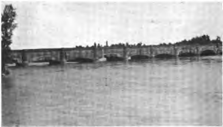
FIG. 135.—Brick Aqueduct, Carrying Cavour Canal, Po Valley, Italy.
